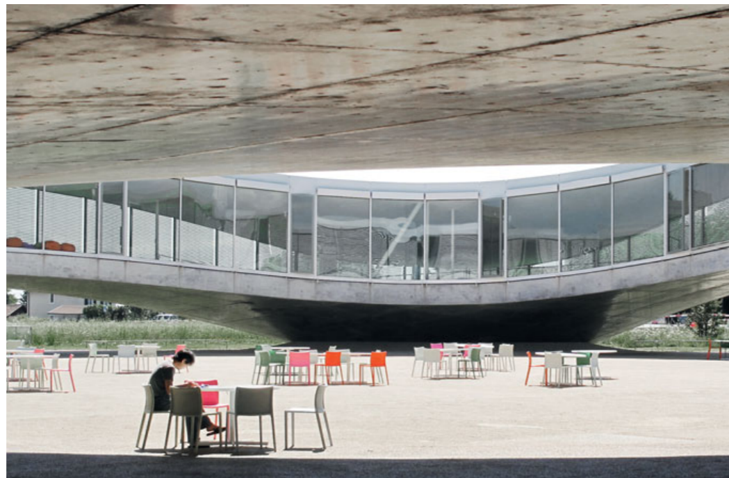
Rolex Learning Centre Lausanne, Switzerland project: Studio SANAA
